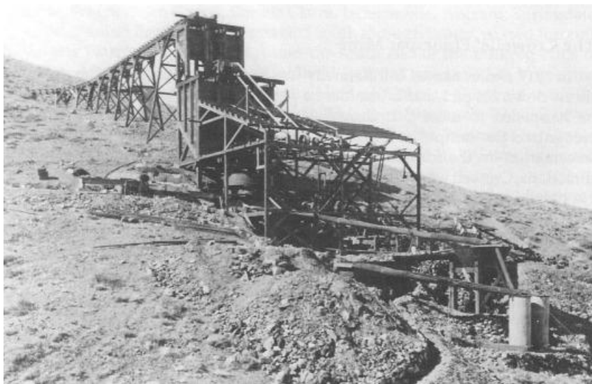
Crowell's mill located at Chloride Cliff in the Funeral Mountains, circa 1915. The mill, under construction, is seen completed in the next photo. It was designed to process ore by the cyanide and amalgamation methods, but only small amounts of ore were ever run through it. - Nye County Town History Projectô Crowell Collection
